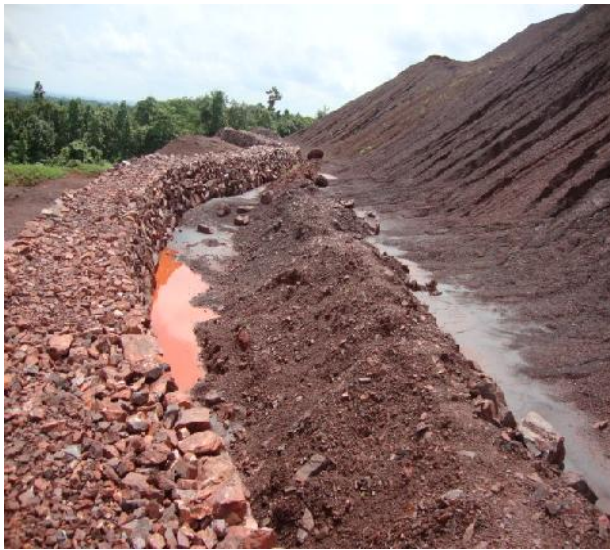
Pic 1- Retaining Wall constructed at the base Of sub-grade dump
