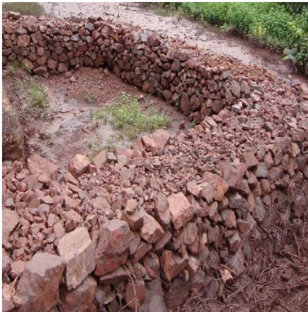
Pic 7- Check weirs near bank of Nallah
