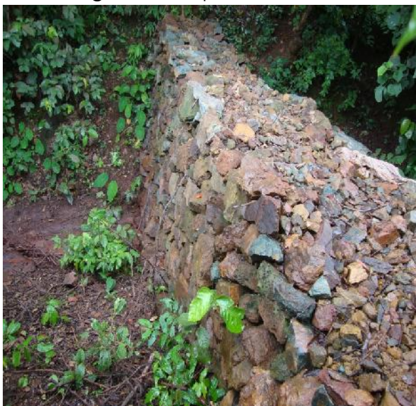
Pic 1- Retaining Wall constructed at the base Of sub-grade dump
